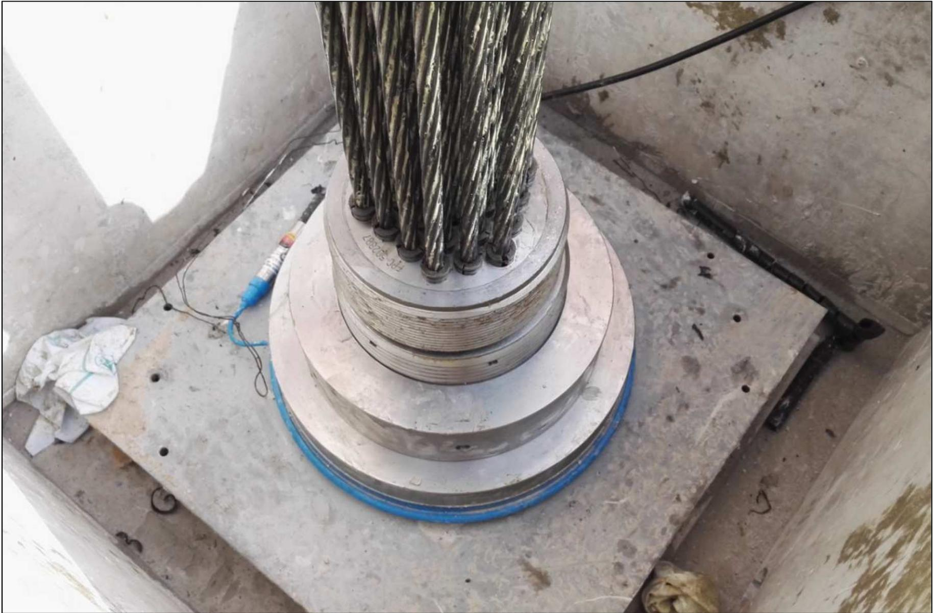
**TETE DE TIRANT TENSION AJUSTABLE EQUIPEE D'UNE CELLULE DE MESURE.**
